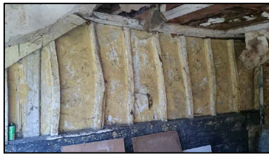
2. Cart House to be reconstructed
