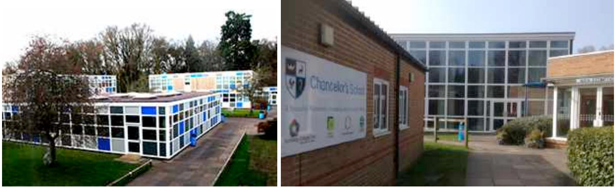
Existing Building Stock at Chancellor's School
