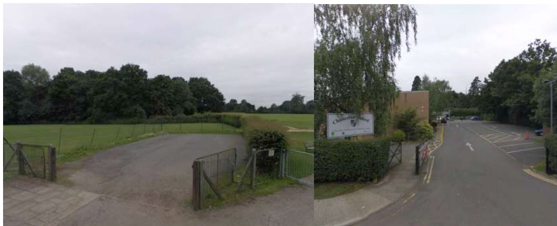
Existing Parking at Chancellor's School
