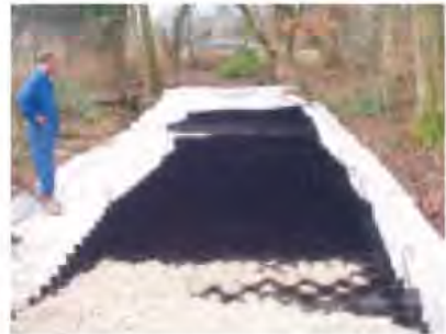
Installation of the CellWeb™ system.
