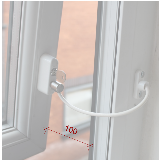
window open showing clear opening of <=100mm PERSPECTIVE VIEW
