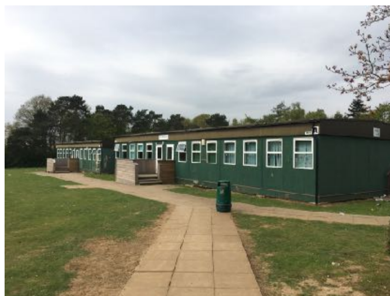
Existing Mobile Classrooms
