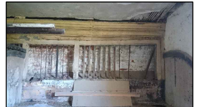
6. Retained moulding feature
