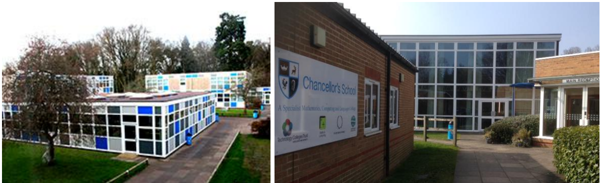
Existing Building Stock at Chancellor's School
