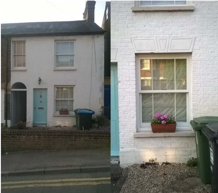
View of the Victorian House with a detailed view of the new window.
