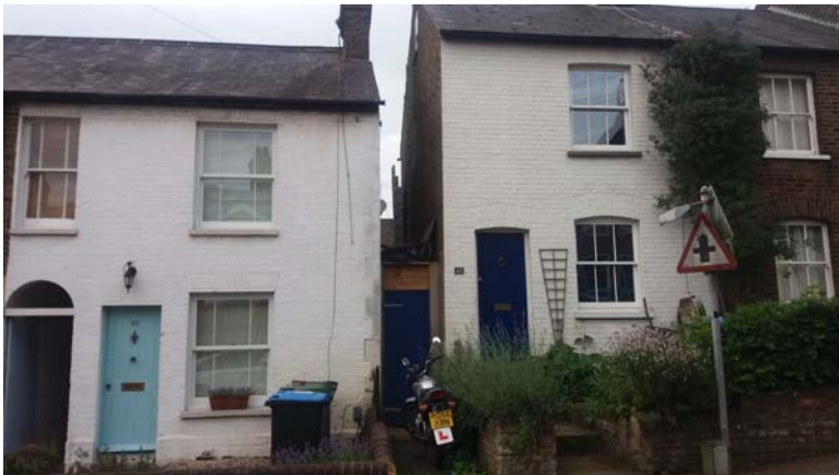
Victorian House - General view of the neighbouring windows and the comparison between new windows and old windows.
