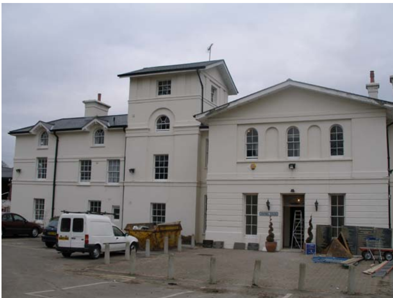
front elevation (south) of Oshwal House
