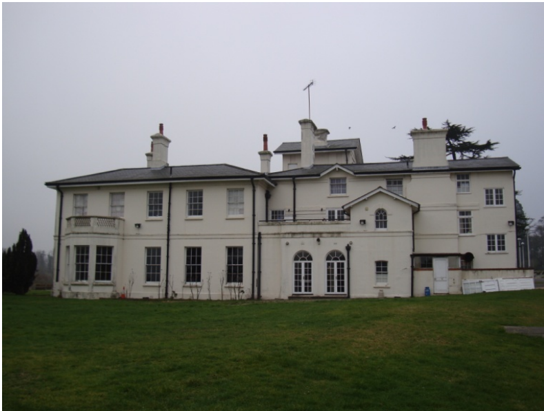
Rear elevation of Oshwal House and the old rear extension to the original House
