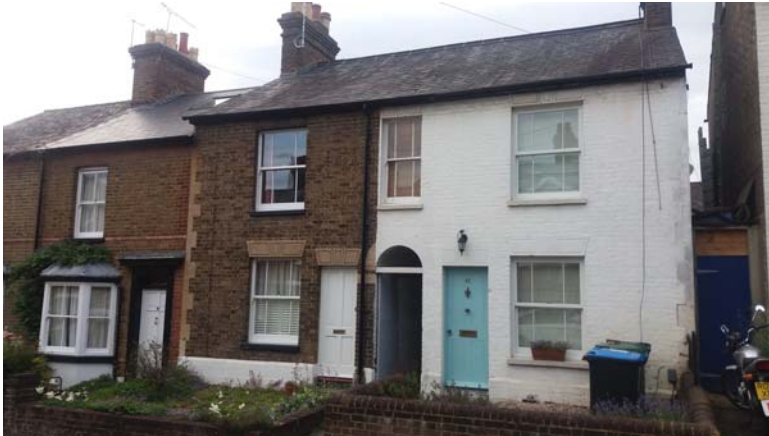
Victorian House - General view of the neighbouring windows and the comparison between new windows and old windows.
