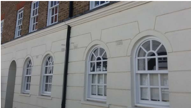
Development in Vauxhall, Detail of the new windows.
