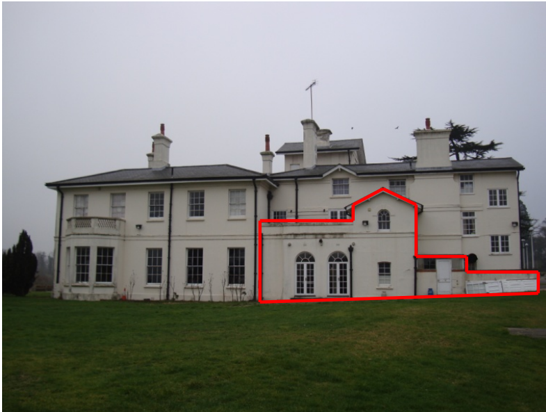
Rear elevation of The Hook House and the old rear extension to the original House
