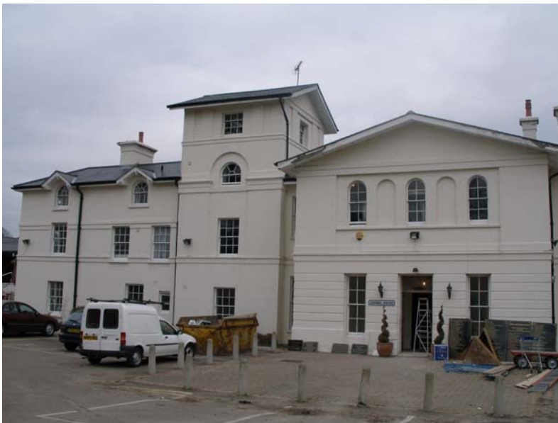
front elevation (south) of The Hook House
