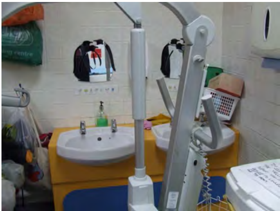
The existing sanitary provisions are currently restricted as specialist equipment is required for the students. Once more there is inadequate storage facilities available.
