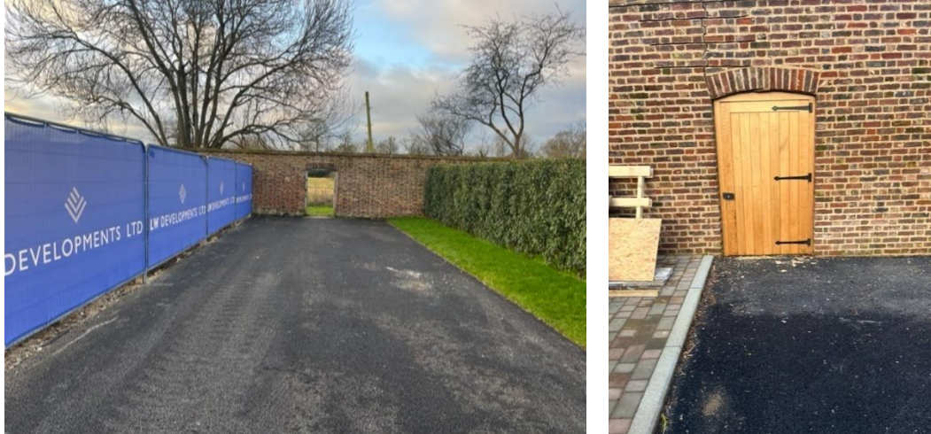
Figures 6 and 7: Existing central access in the southern wall (left) and existing opening within the walled garden serving Oak Cottage (right), the detailing of which will be replicated by the proposed openings
