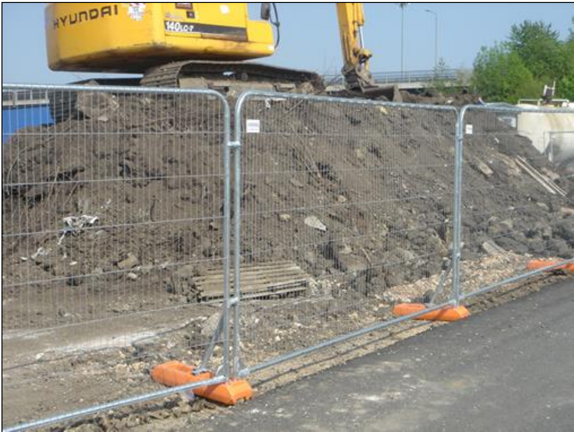
Photograph E – Example of Heras Tree Protective Fencing
