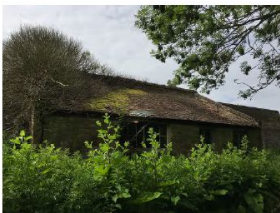
Plate 31: Building 2: Brick Gardener's Store as seen from the north
