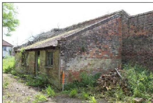
Photo 147: Overview of western and northern elevations of Outbuilding 2
