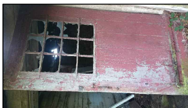
3. Yard doors to be preserved and re located in front of the original position
