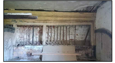
6. Retained moulding feature
