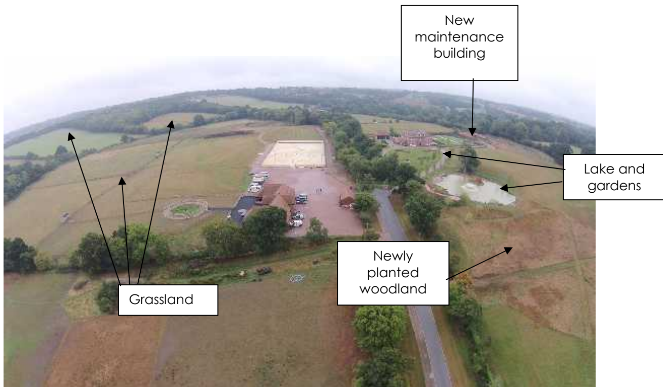
An aerial view of the site
