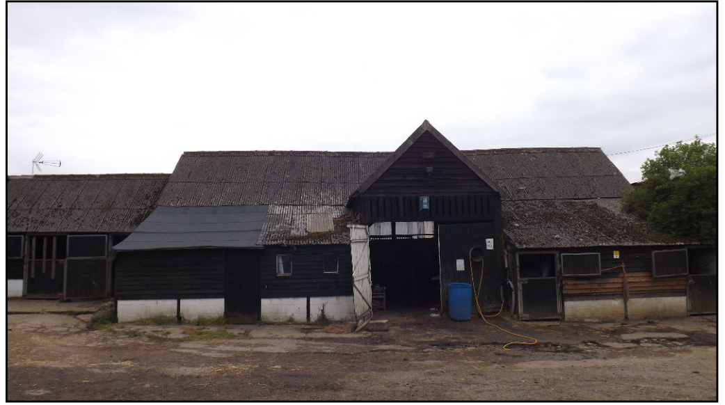
B. Barn (3) west frontage
