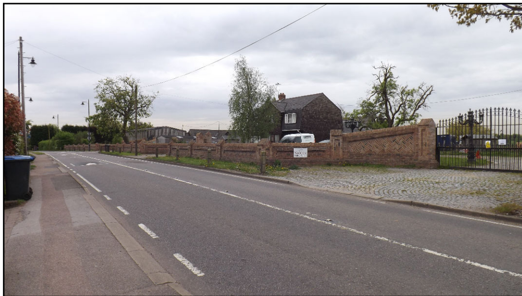
C. Front wall and house, looking south-east
