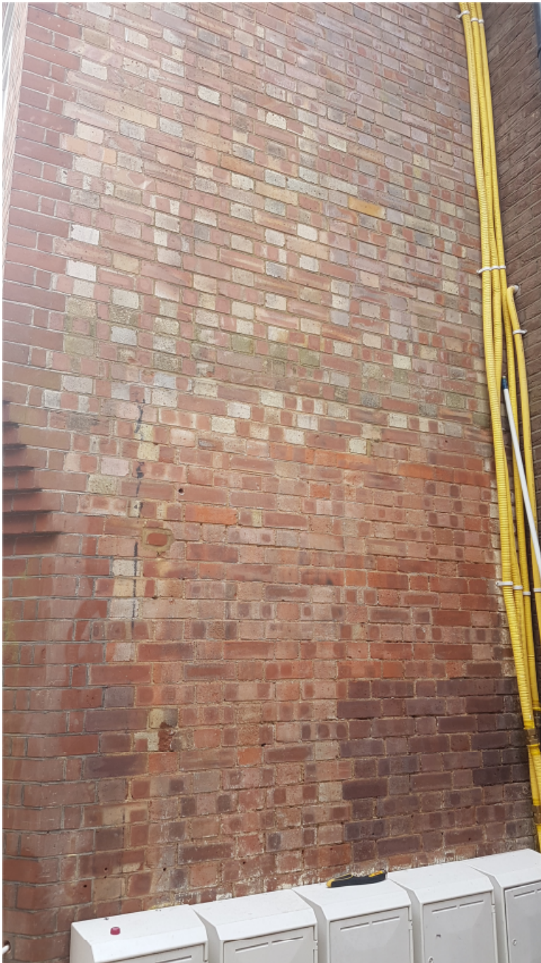
Elevation with existing Common Bricks (Before treatment)
