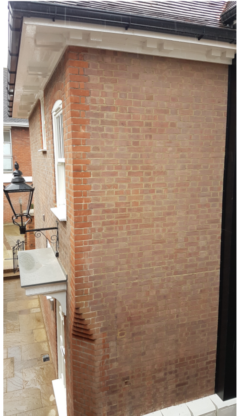
Same elevation following re-pointing and surface treatment (After treatment)
