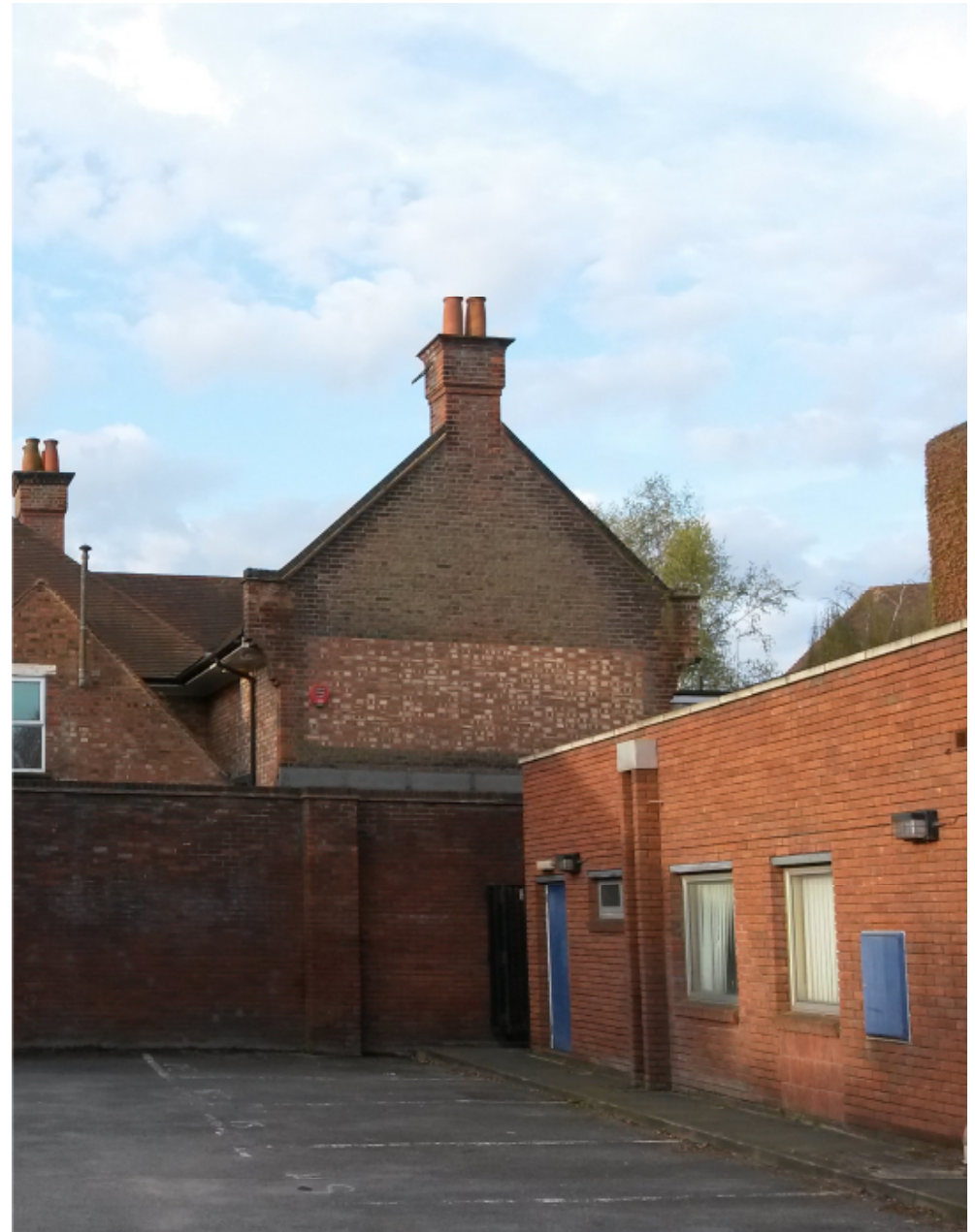
Rear elevation showing inset of common bricks (Before Brick Treatment)
