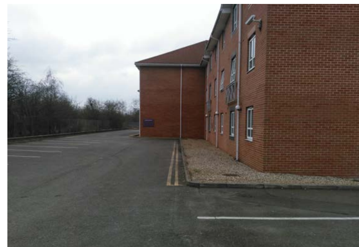
View south towards boundary with railway line
