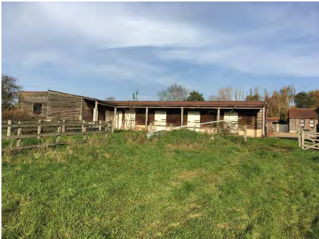
Plate 6. Modern stable block adjacent to the paddock to the south-west of the yard, looking north-east
