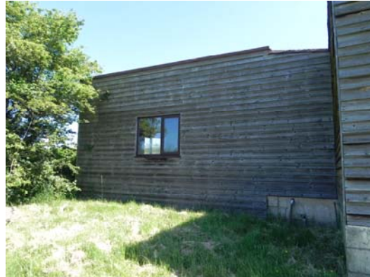
Photograph 26: end storage unit
