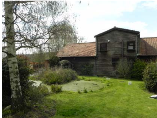
Photograph 9: office northeast elevation
