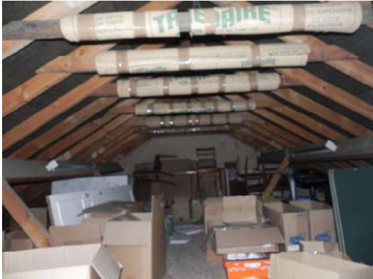
Photograph 11-12: office southeast loft structure
