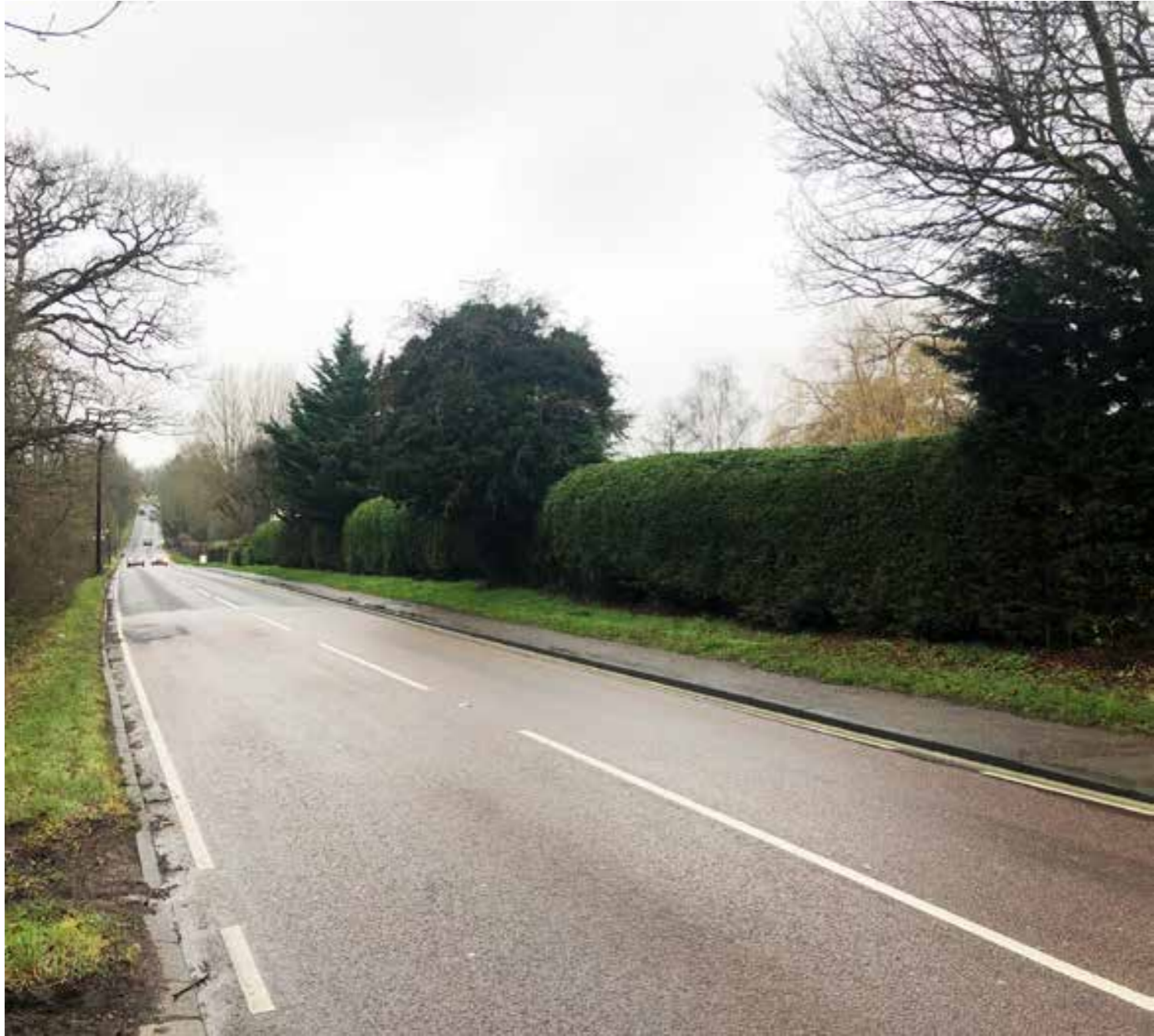
Existing view looking west down Northhaw Road East from the field access opposite the Football Club.
