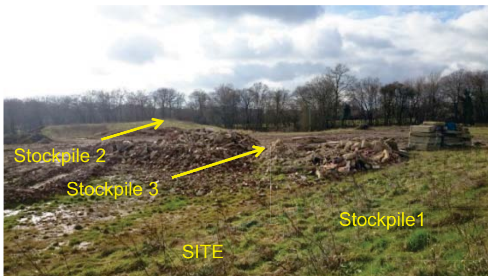
View south-westwards across the site, showing the three stockpiles.
