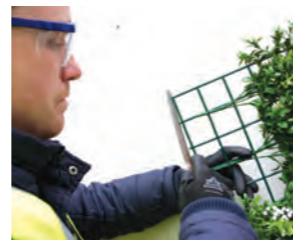
Step 3 File the grid after cutting.
