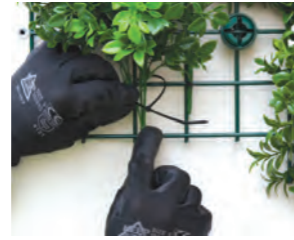
Step 5 Re-attach loose from the vertical off-cuts with cable ties.
