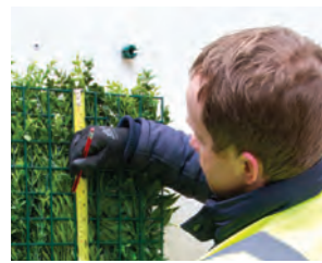
Step 1 Measure carefully and mark the area to be trimmed.
