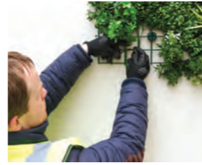
Step 6 Re-adjust any plants on the cut parts and fill in all the gaps with loose foliage in the horizontal cuts.
