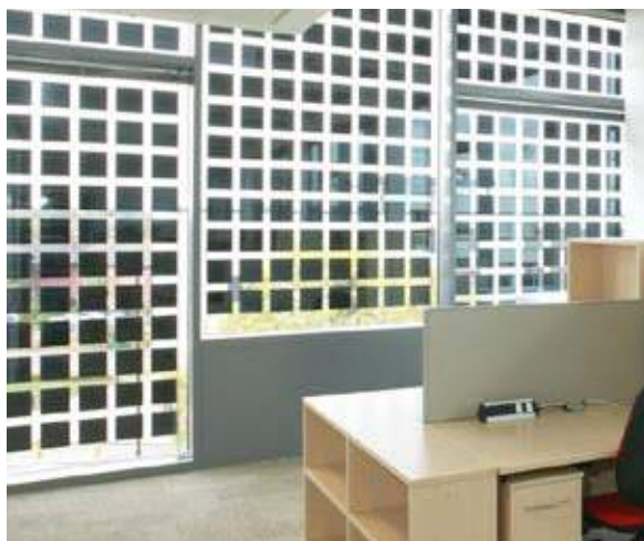
CPW Solar Glazing Installation, University of Warwick
