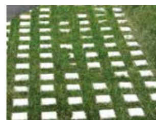
Type of reinforcement to grass
