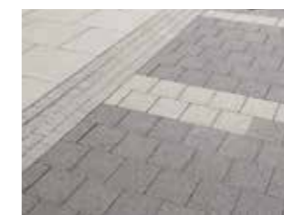
High quality Slab/ Block paving
