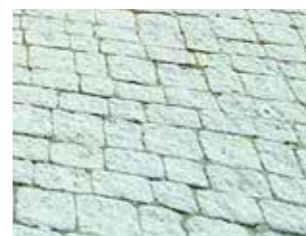
Sett paving to match existing
