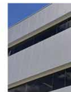
2. Metal Cladding Panels
