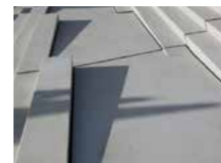
Feature concrete steps & seating
