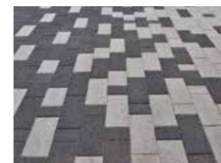
Transition zone - 2 types of paving
