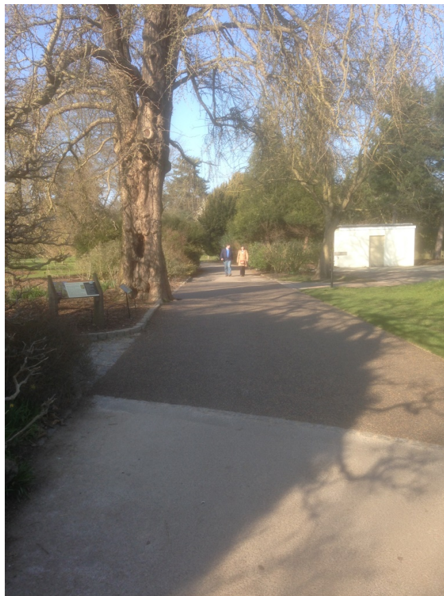
Kew Gardens (London): Resin Bonded Gravel used across a root-plate of the TROBI Champion Ginkgo
