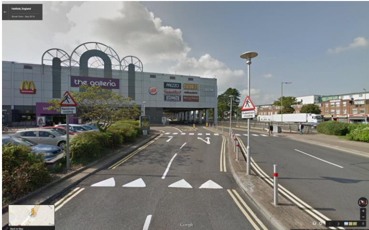
Figure 2: Speed hump and zebra crossing
