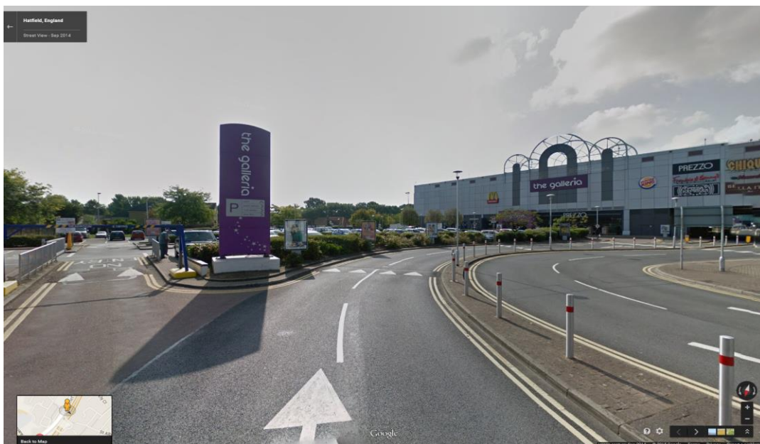
Figure 1: Existing Entrance Road Layout from the North
