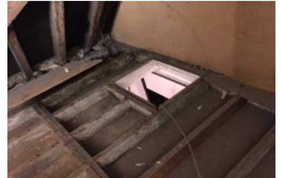
Formed roof hatch of 20 th century
