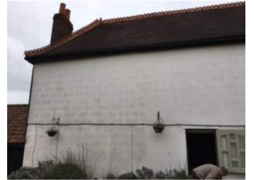
Note the blockwork elevation to courtyard of unit 2
