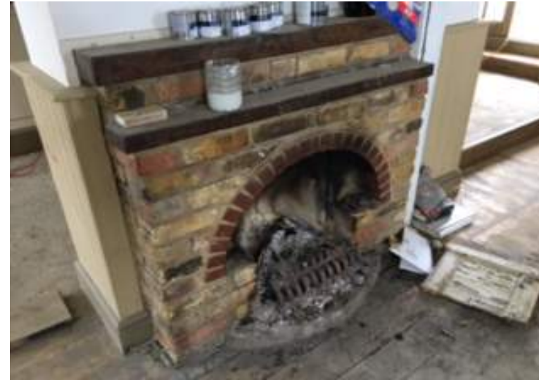
Dual fireplace to unit 2 bar area
