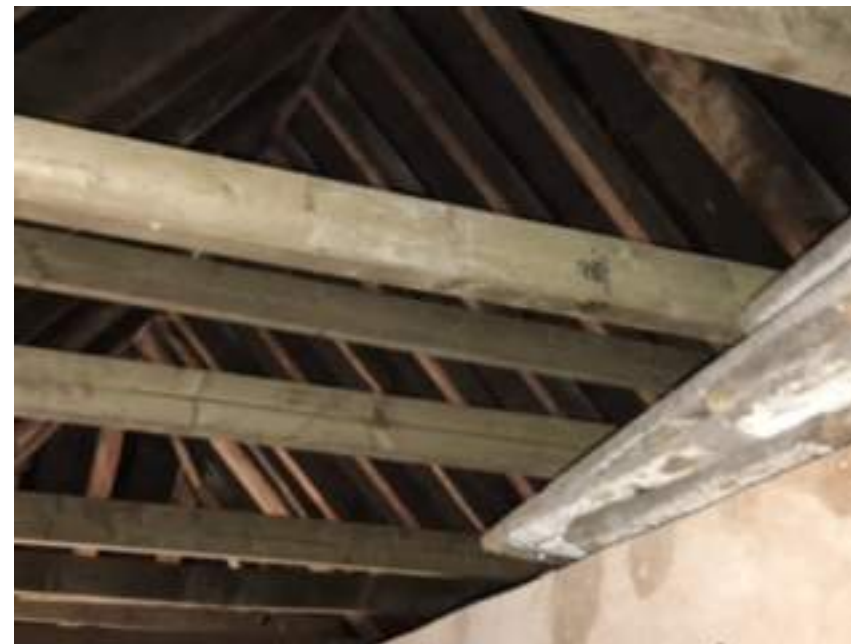
Modern sawn timber to ceiling of unit 1
