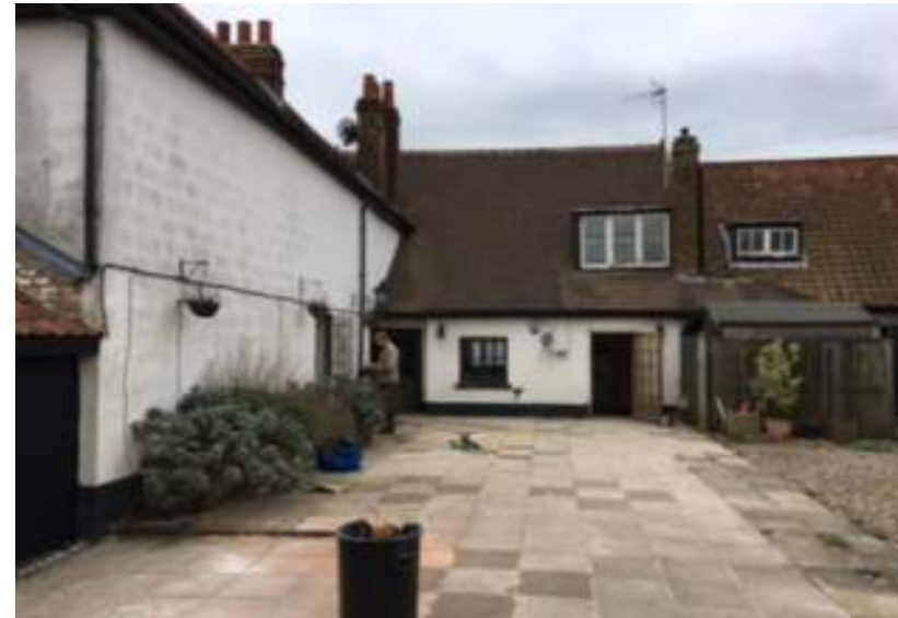
External courtyard areas.
