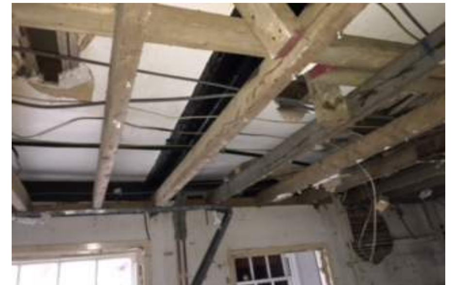
Original floor joist above suspended ceiling.
