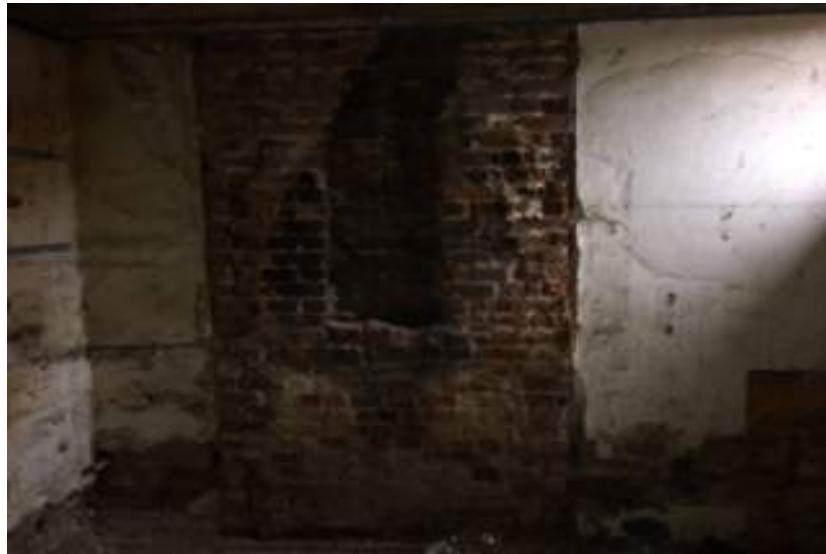
Unit 1 chimney breast remains
