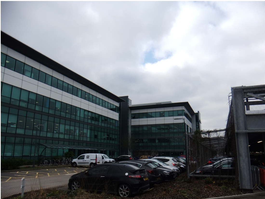
Fig 2b. Photograph of host building,
