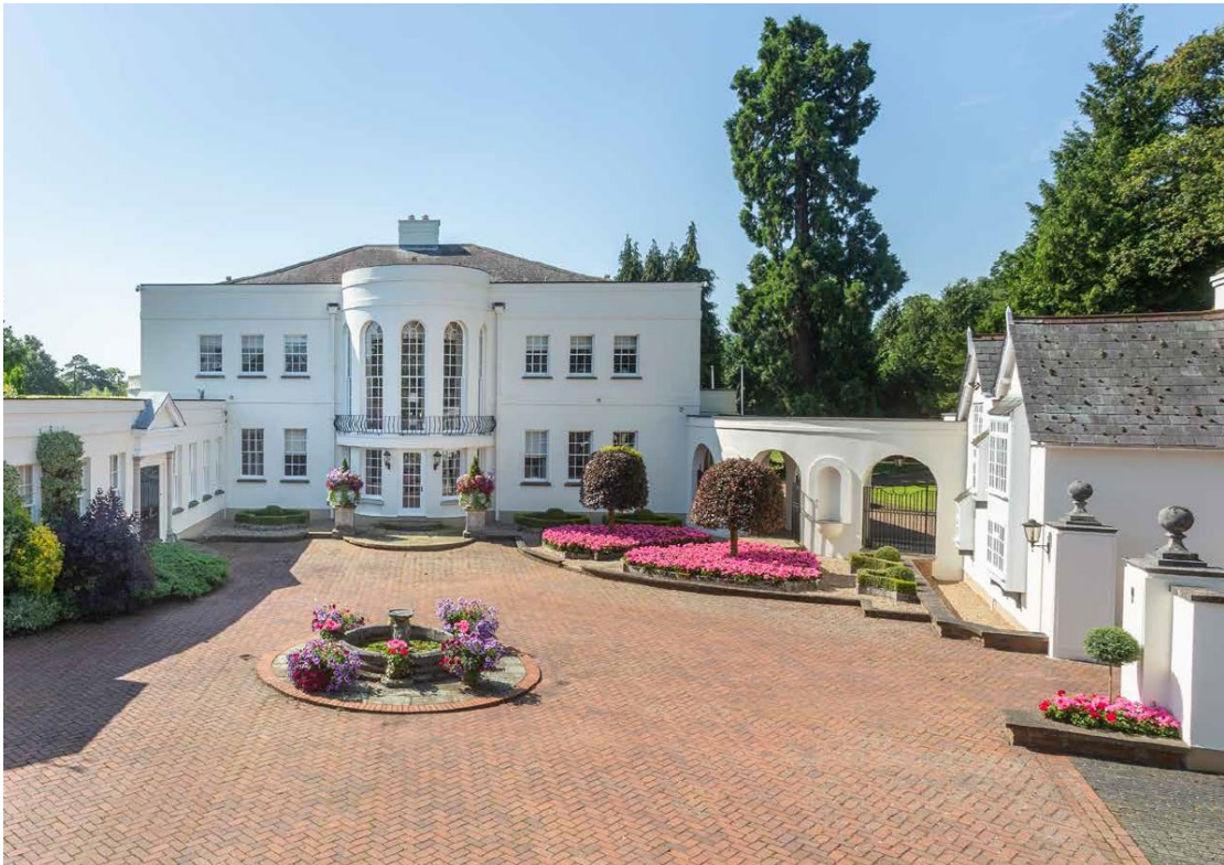
[The north elevation of the existing dwellinghouse together with the attached guest suite and part of the adjacent internal courtyard. Photograph courtesy of the recent sales particulars produced by Savills and Strutt & Parker]
