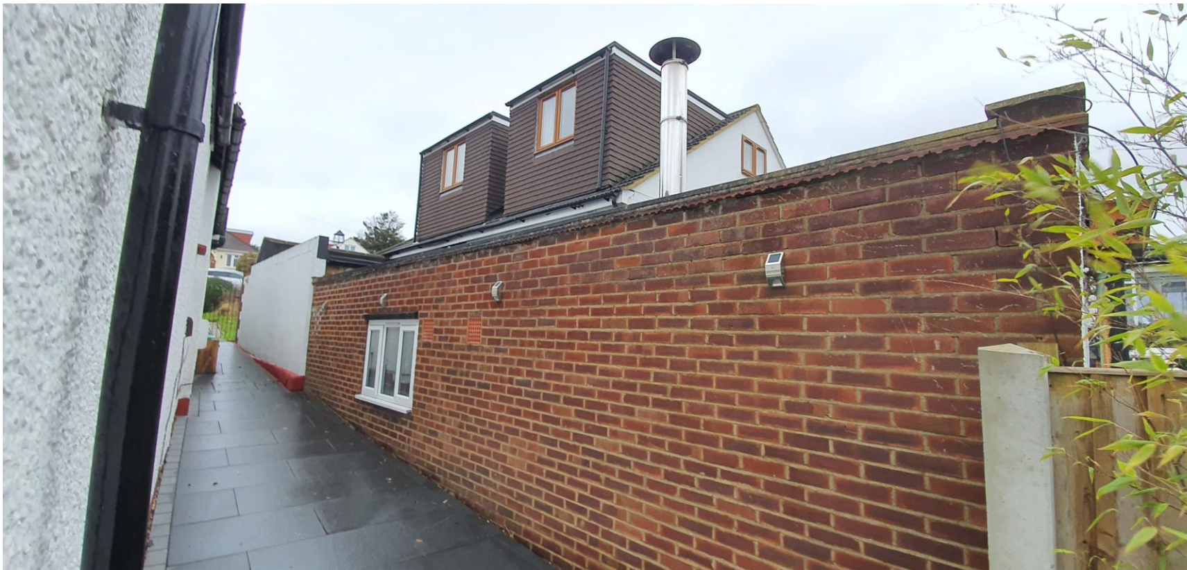
View from Rear Side entrance showing No.33
