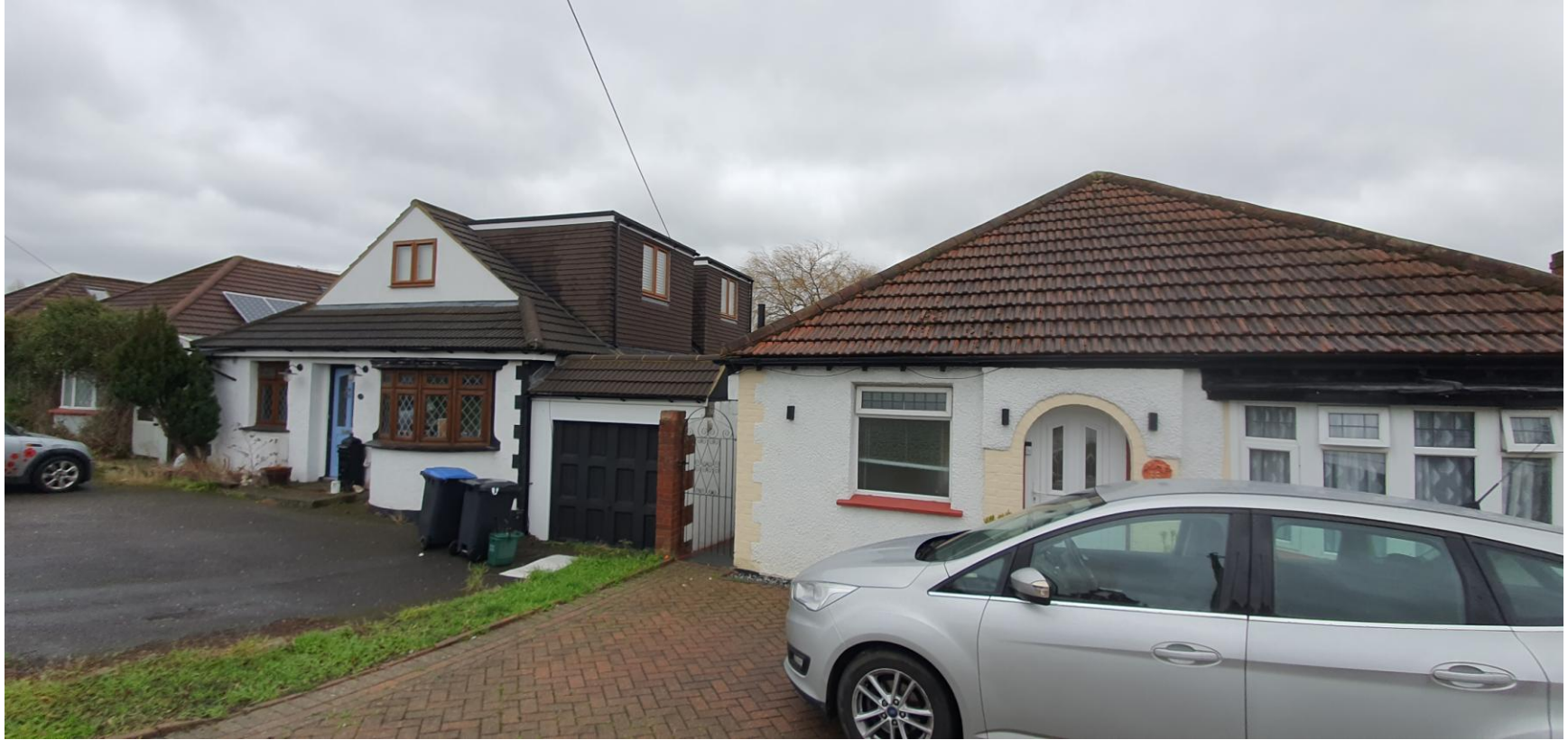
Front View towards No.33
