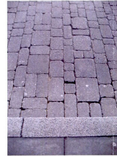
'Conservation' kerb & Granite sett paving
