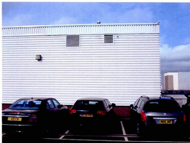
PHOTO OF SIGN LOCATION
