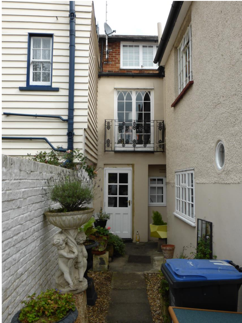
1. Rear Elevation (Looking into Recess).
