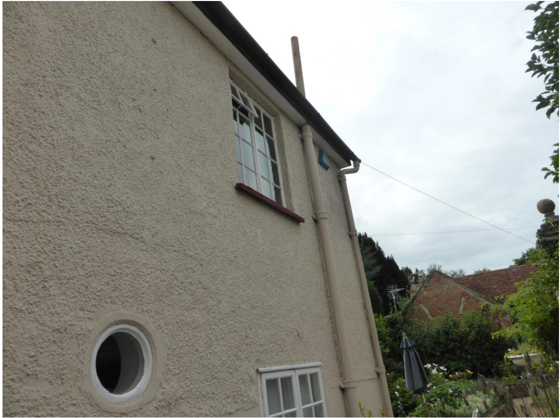
9. Window to dressing room.
