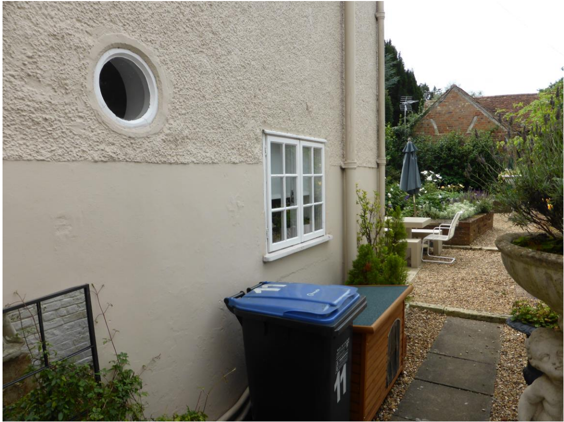
7. Kitchen window to rear of addition.
