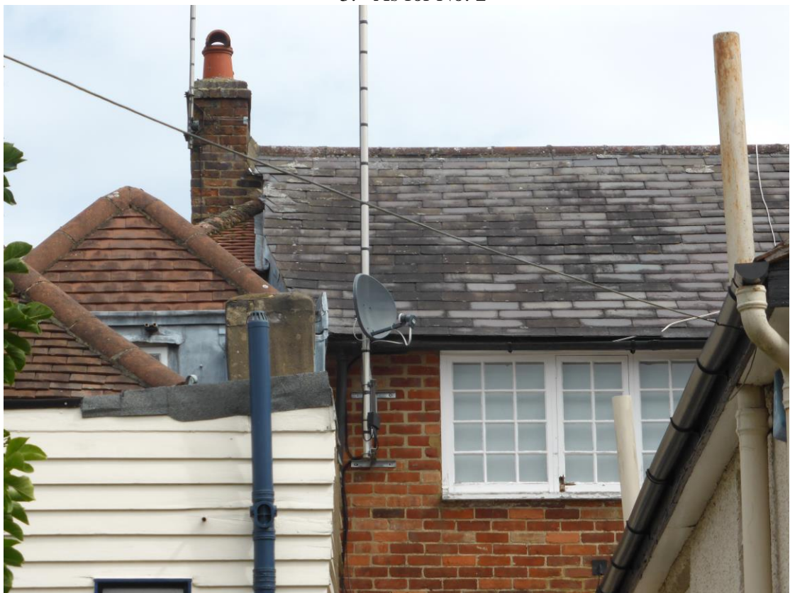
4. Top landing window to main rear elevation.
