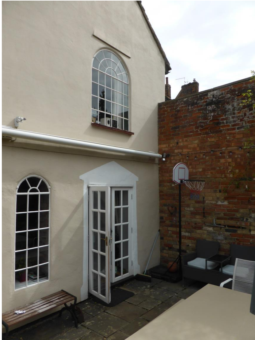
2. Rear Elevation of two storey addition.
