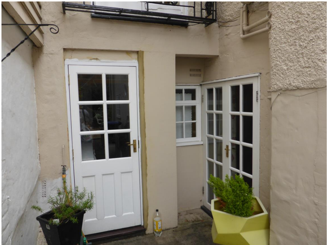
6. Rear doors and window within recess.
