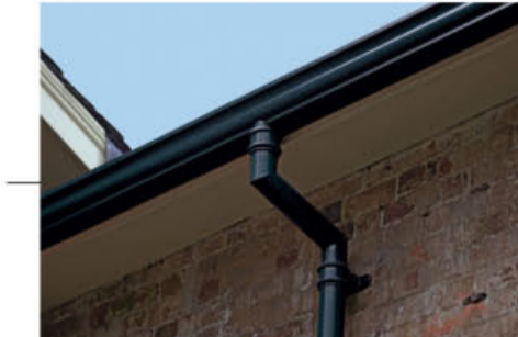
BLACK UPVC GUTTERS AND DOWNPIPES
