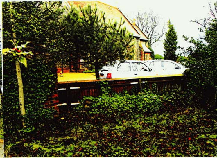
Temporary timber fence for security where existing wall has collapsed
