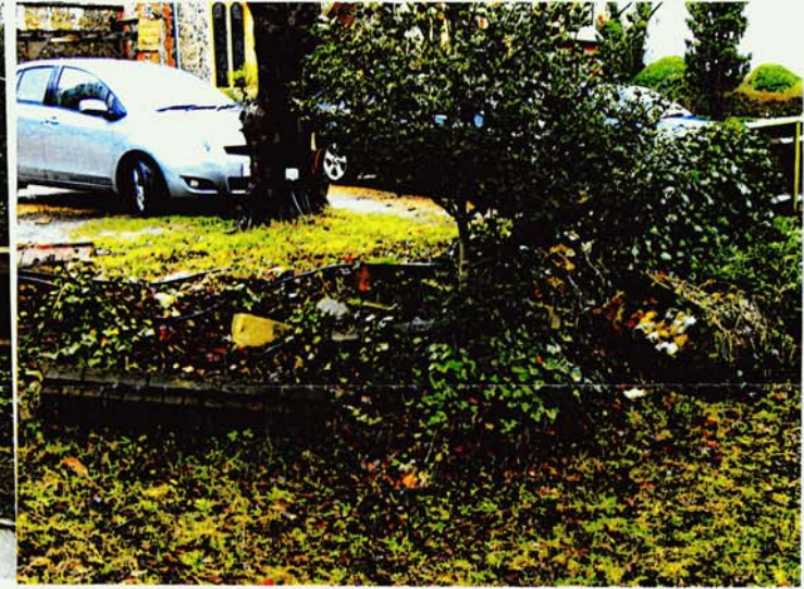
Materials from collapsed wall to be reused.
