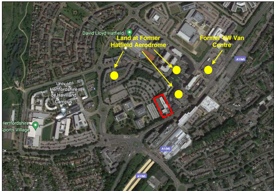
Figure 7: Map showing the location of relevant planning applications in the surrounding area
