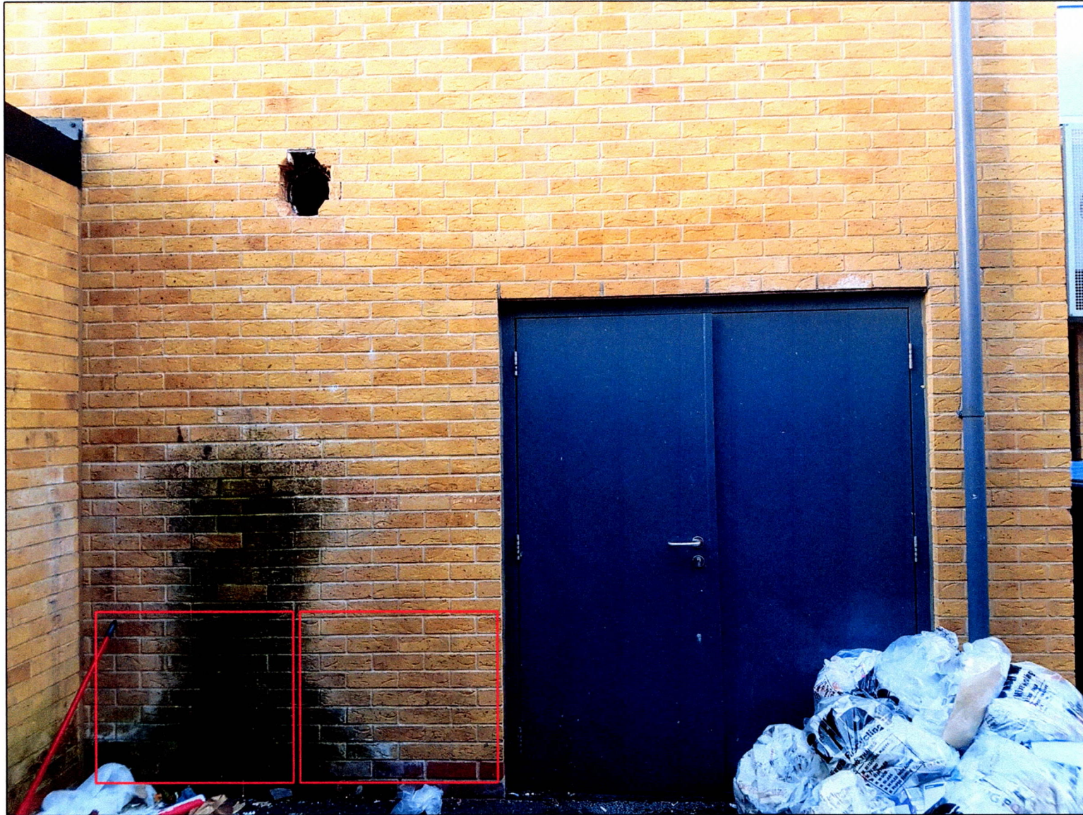
The red box is a rough indicator of where the condensing units will be placed.
