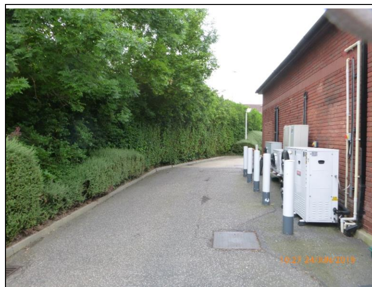
E View looking south behind the shop.
