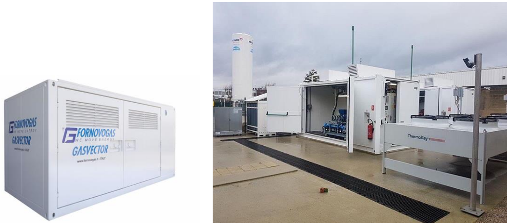
Figure 3.2.1. – Compressor Housing
