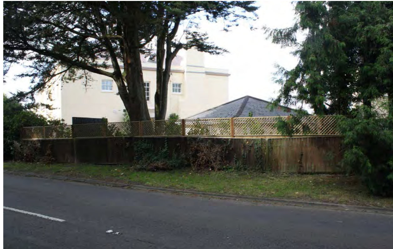
Photograph I View of building towards Dimsdale House on western side of High Road
