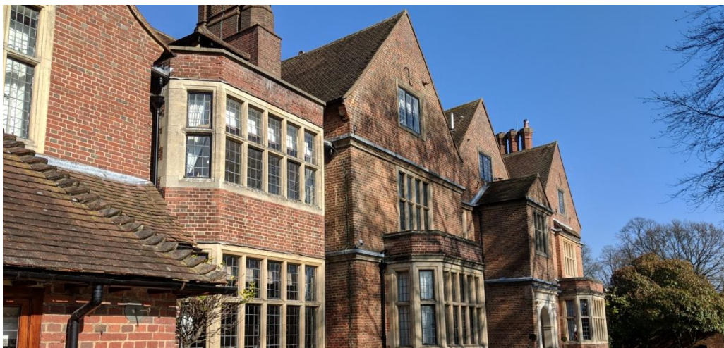
figure 2: Close-up view of North Elevation
