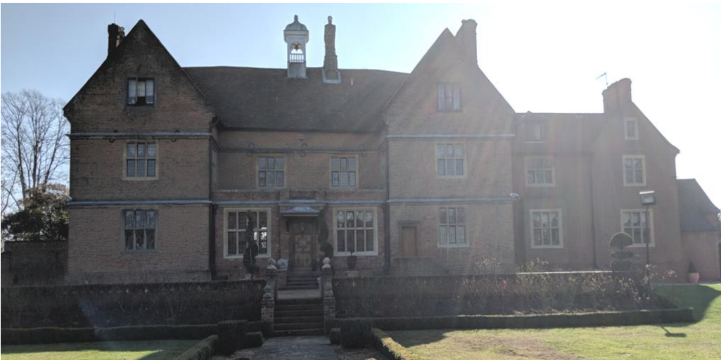
figure 4: View of South Elevation
