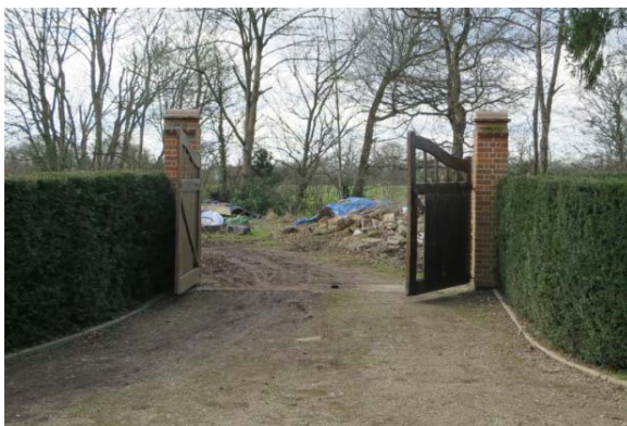
IMAGE 7: Existing gate to be replaced.
