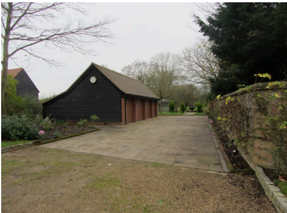
Site of newly completed garages outside of wall enclosing proposed site.
