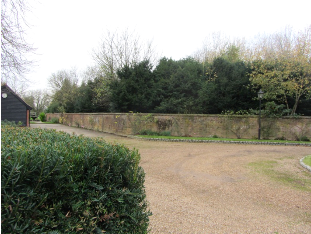
View of existing wall (2m high) from outside proposed site.
