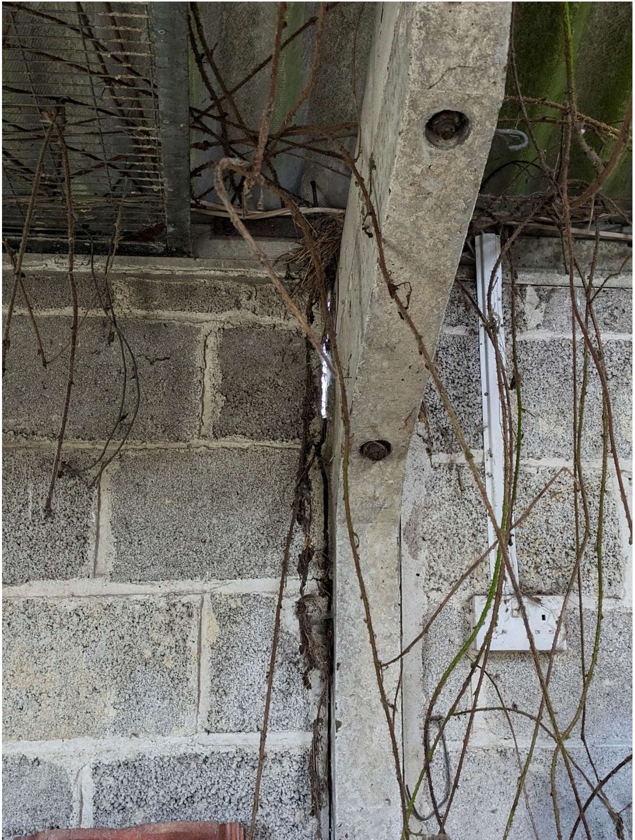
Photograph 4 Typical view on infill blockwork to external leaf.
