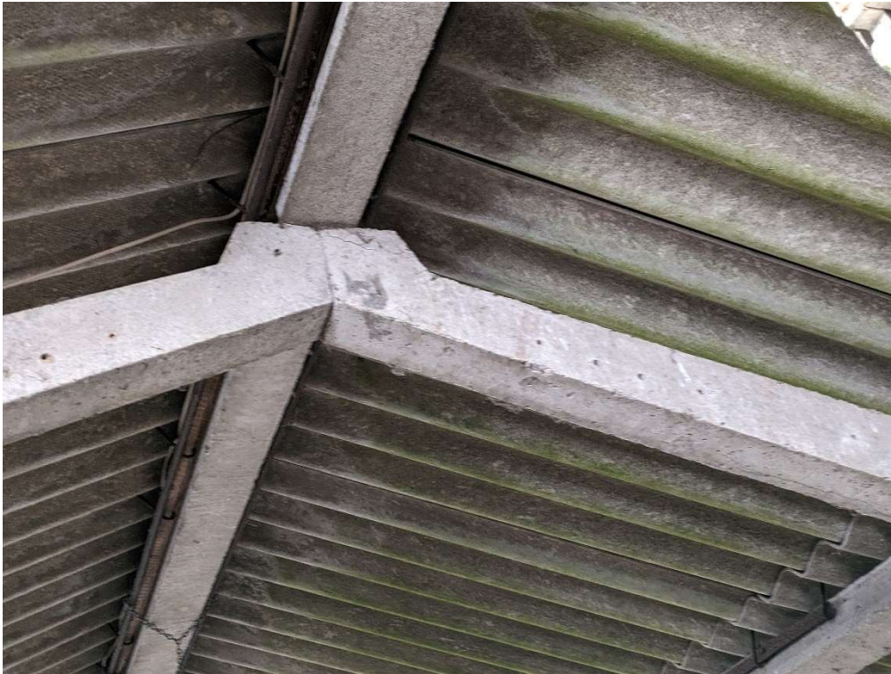
Photograph 6 View on precast concrete ridge beam.
