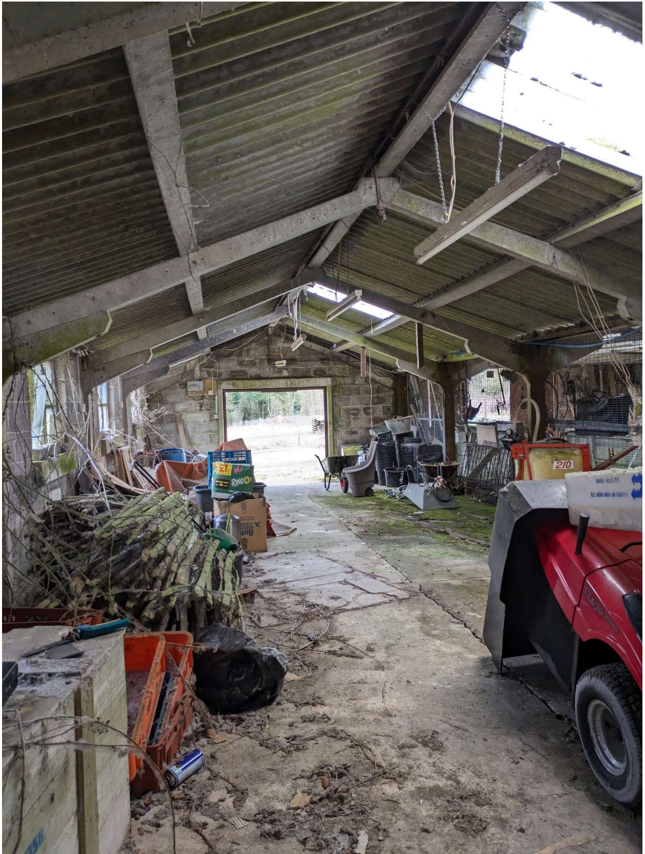
Photograph 2 View on one half of double portal frame.
