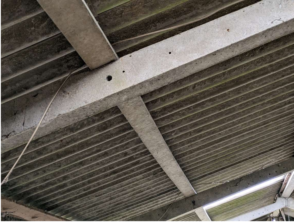
Photograph 7 View on precast concrete purlin.
