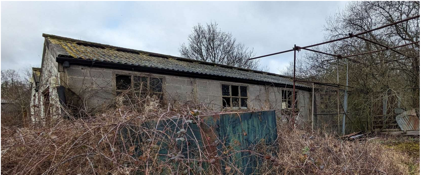
Photograph 10 View on right hand side external elevation.
