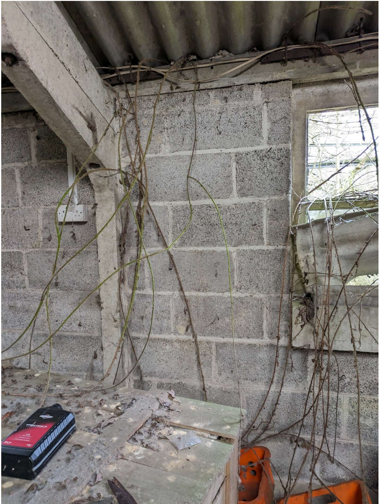
Photograph 3 Typical view on infill blockwork to external leaf.
