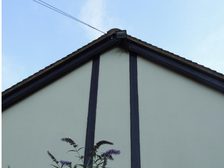
Photo 15: Note tight seal to gable
