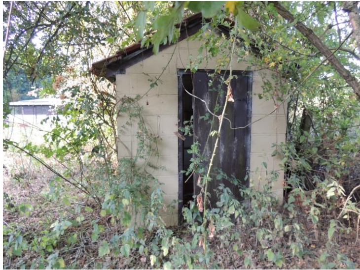
Photo 21: Small toilet building
