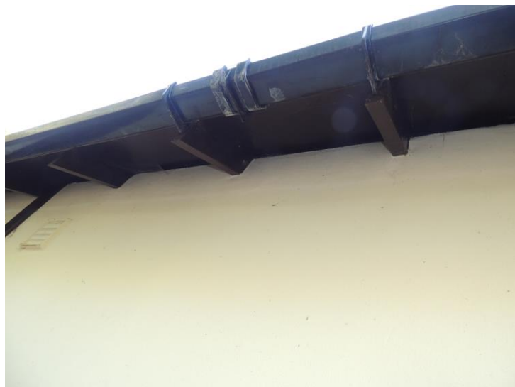
Photo 16: Typical section of eaves showing tight seal
