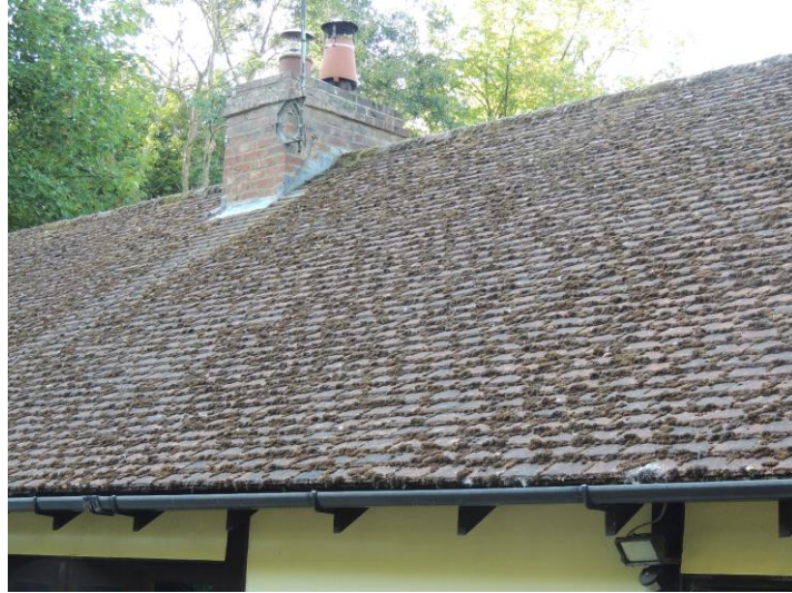
Photo 18: Note tight seal to roof tiles
