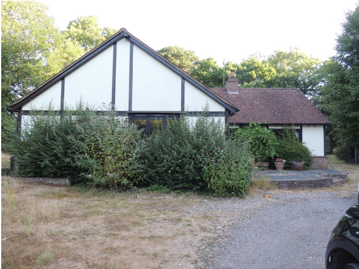
Photo 1: Front (southern) elevation. The proposal is to demolish and replace the building
