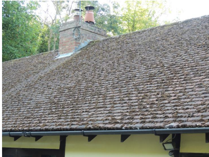
Photo 18: Note tight seal to roof tiles
