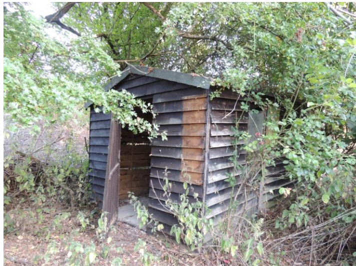
Photo 19: Wooden shed due to be demolished
