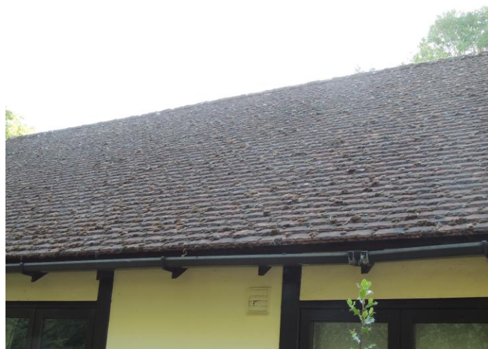
Photo 17: Note tight seal to roof tiles
