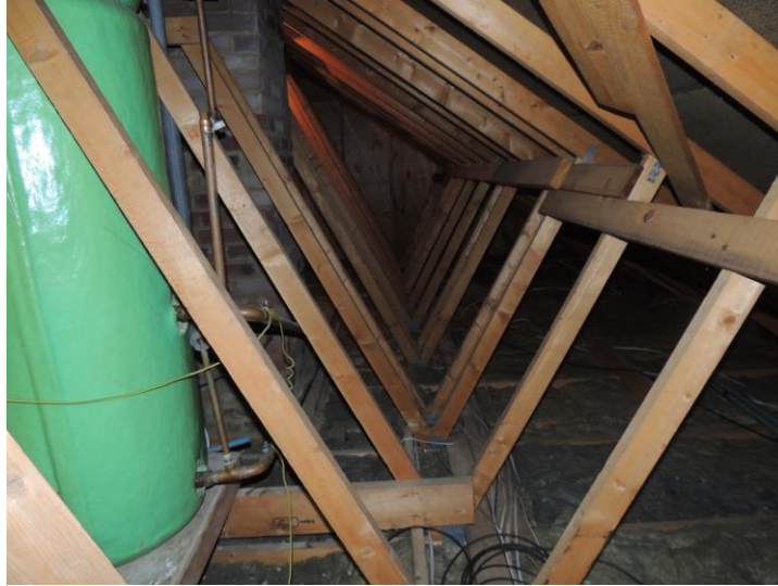
Photo 12: Note trussed roof construction
